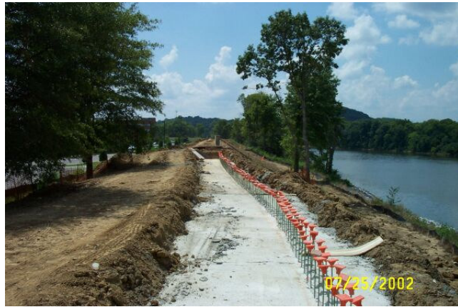
Figure 4-6. Metro Center Levee Rehabilitation
