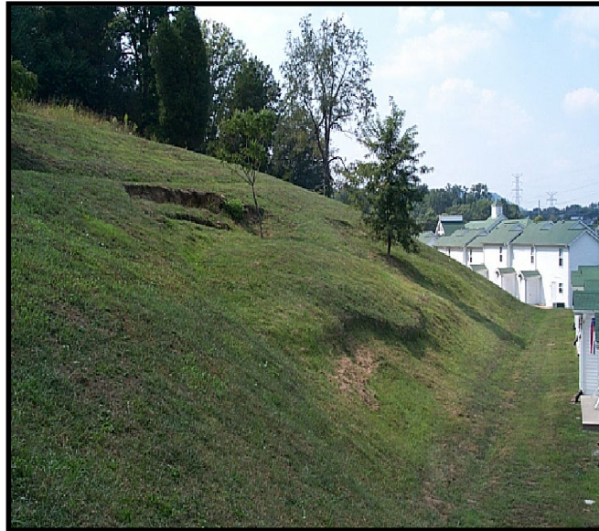
Figure 4-10. Evidence of Landslides
